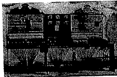
An Early PBX This PBX began operation in Bangor, Maine in 1883. (Image courtesy of AT&T.)
