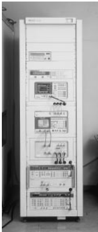
PHS custom test system
