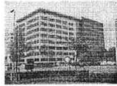
Le Croisé Building
