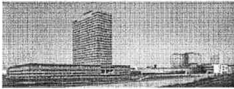
Tower, Hinge and Shell Buildings
