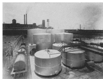
Tank Farm and filling equipment
