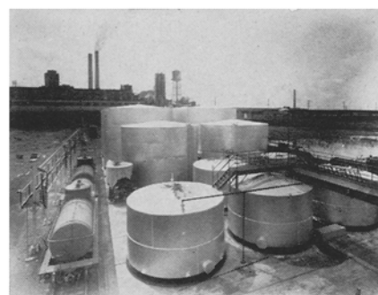
Tank Farm and filling equipment
