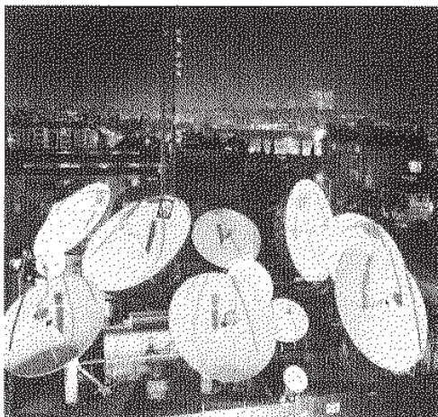
FIGURE 11.14 Many syndicators use satellites to feed programming to client stations. This greatly simplifies the distribution process. Handling of tapes and mailing is eliminated. Satellite syndication also keeps station equipment costs down. Courtesy IDB.
